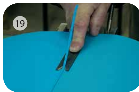
Using V-trimmer to trim excess from weld
