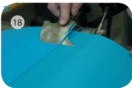
Using Leister Knife to trim excess from weld
